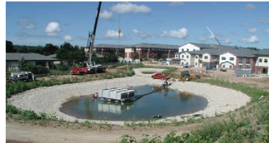
200 Ton SLIM JIM® Project—Wisconsin—Installation
