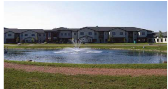
200 Ton SLIM JIM® Project—Wisconsin—Complete
